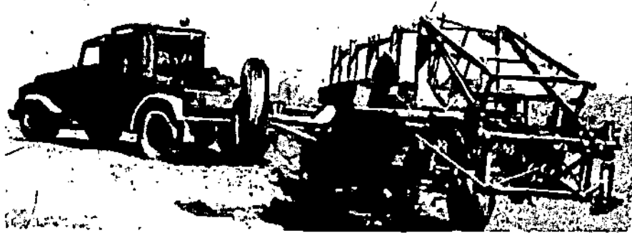
Lock Carriage Securely Before Transporting.
