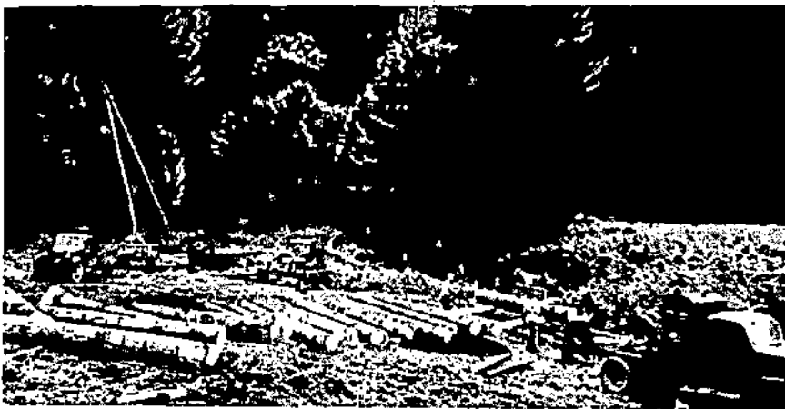
Build Skidway on a Gradual Slope.
